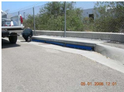
During fiscal year 2007-08 the BioClean filter that was installed on the 12” pipe that discharges to Oceanside Blvd was removed due to constant clogging and replaced with fiber rolls around the inlet. This drainage area will be checked regularly to remove debris collected around the fiber rolls and to ensure that the fiber rolls in proper working order.
