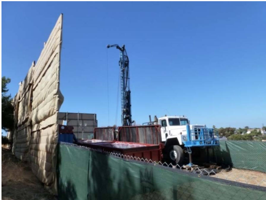
Figure 4 Curtain-Type Noise Barrier
