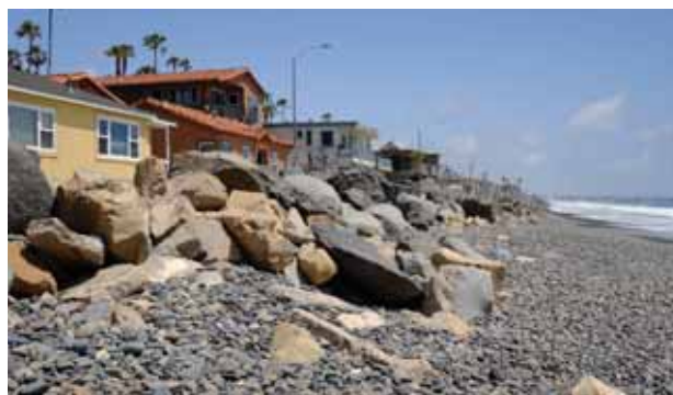
An existing rock revetment along The Strand
