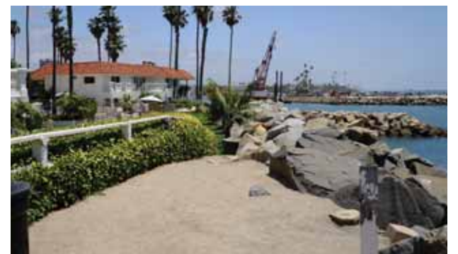
Rock revetments in the harbor protect inland properties
