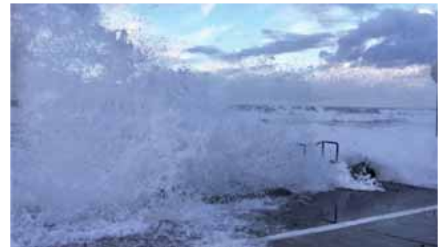
Walls and revetments can be overtopped during storm events
