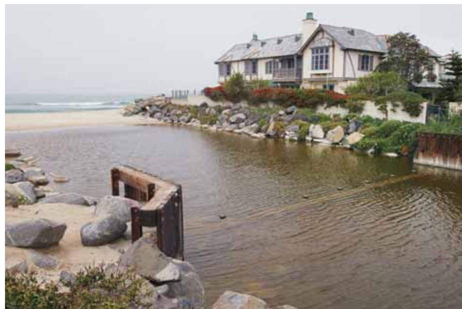
The weir at Buena Vista lagoon
