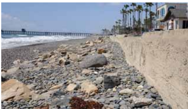
The existing sea wall along The Strand
